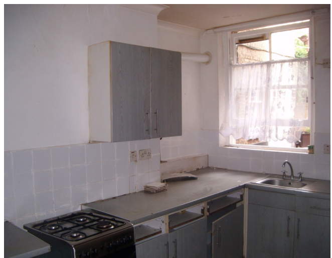
Kitchen before upgrading
